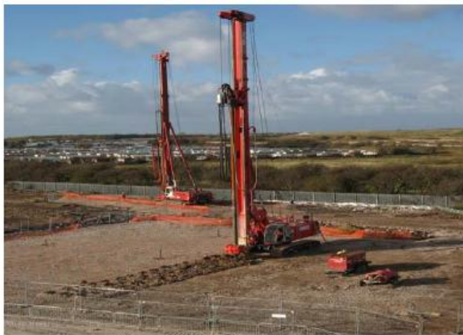
Figure 1: CFA Rigs In full swing
