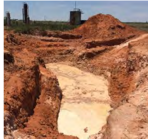
Wet mixing completed.
