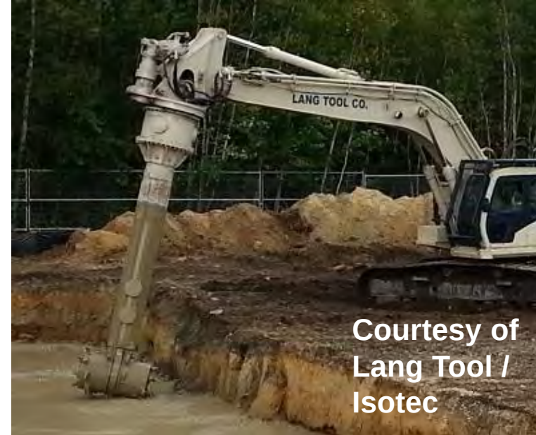
Soil mixing using excavator with mixing attachment
