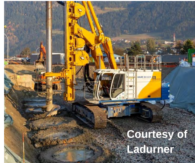
Soil mixing using large diameter augers
