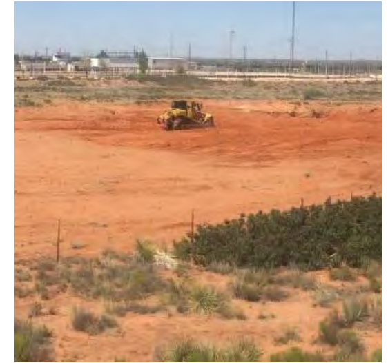
Area after backfill.
