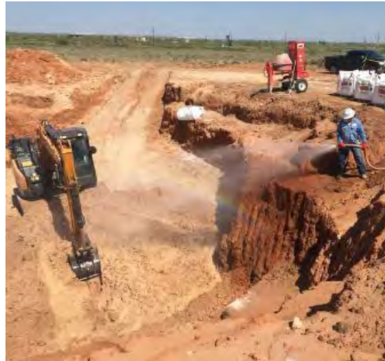
Blending & addition of water.
