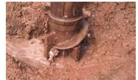
Figure 2. Magnets, within protective latex glove, placed within coring returns on A-6.
