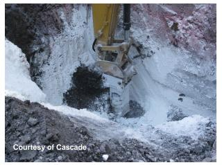
Design considerations are site specific. Among the most critical design parameters are the loading rates of the different reagents to be added. Loadings can vary both horizontally from cell to cell or column to column or vertically if using a mixing technology that allows placement of the reagents at depth.
