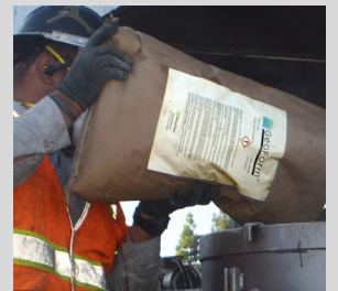
Figure 2. Addition of GeoForm Soluble Mix to mixing tank
