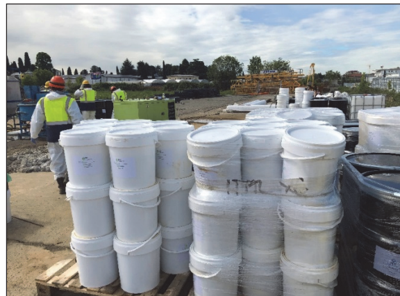
Fig. 6. ELS® Microemulsion component in 200 L steel drums, and EHC® Liquid mix component in 11.7 kg bags delivered in plastic pails
