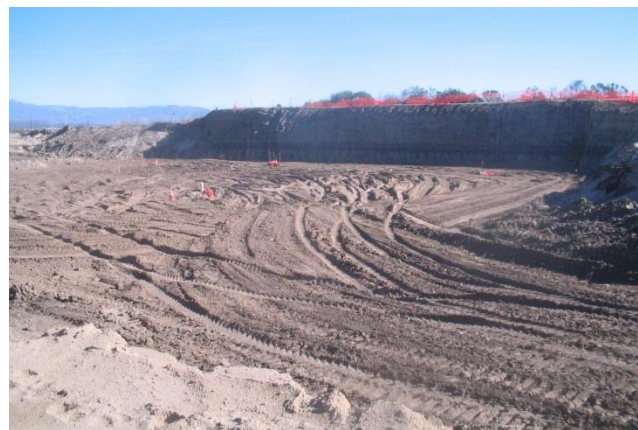
Backfilled 'right eye'
