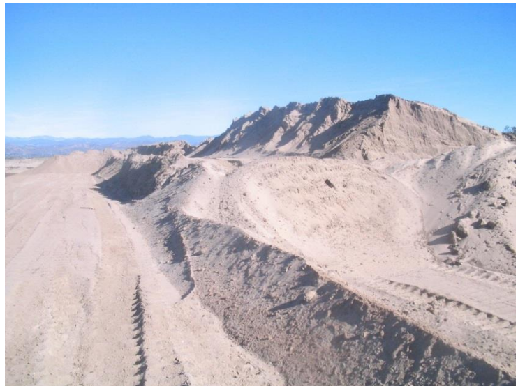
Stockpile of Daramend - sand mixture
