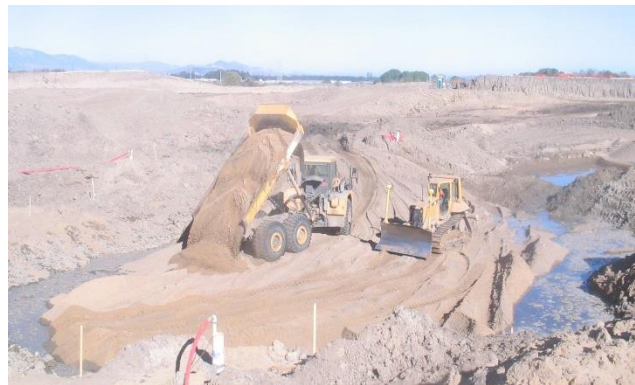
Backfilling excavation
