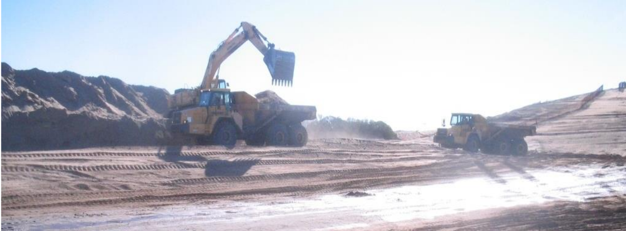
Loading Daramend-sand mixture from the stockpile
