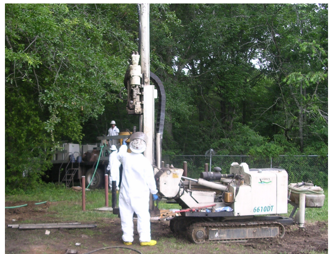
Figure 1. Application of EHC Reagent slurry using direct injection
