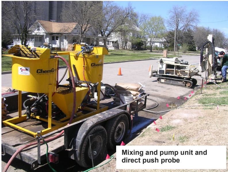
Figure 3. Injection set-up and soil verification borings
