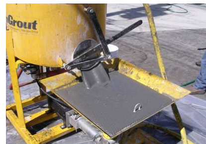
Figure 1. EHC Slurry for DPT Injection
