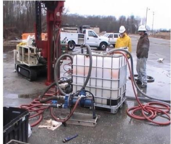
Figure 3: EHC Liquid Injection Preparation
