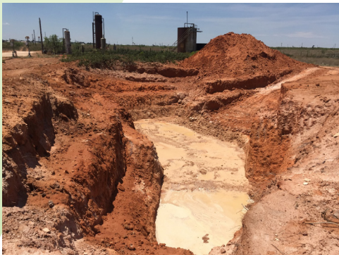
Figure 4. Vent Excavation after Completion of Wet Mixing
