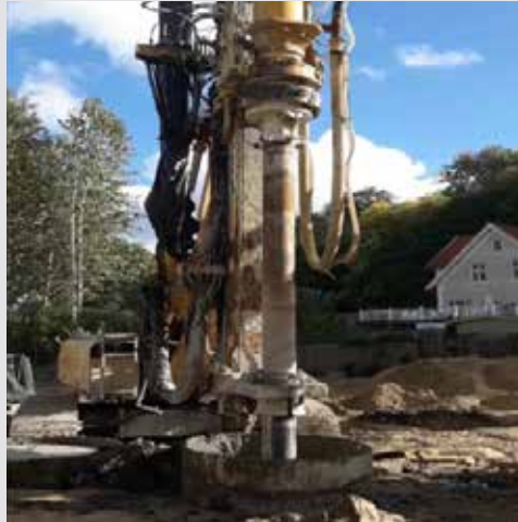
Figure 3. Drill rig 100 ton RTG machine RS20.
