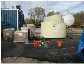
Use of sodium hydroxide (caustic) provided the high pH activation of sodium persulfate. High pH activation was selected as the optimal ISCO technology because of its treatment effectiveness on both chlorinated and petroleum hydrocarbons, the rapid cleanup timeframe, and its relative low cost application.
