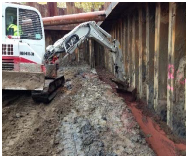
Figure 3. Installation of MetaFix PRB
