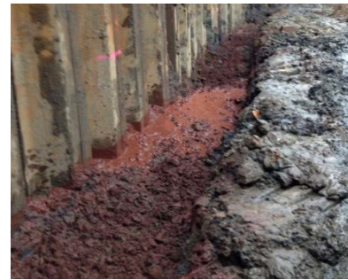
Figure 4. MetaFix reagents blended in to backfill soil
