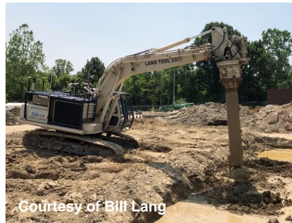
Soil mixing using specialized tools
