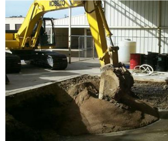
Soil mixing using buckets
