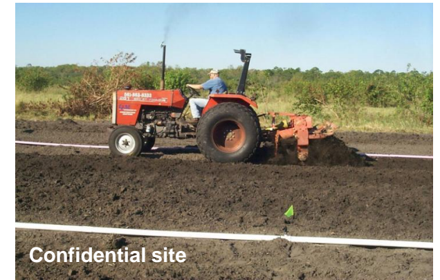
Soil mixing using tillers
