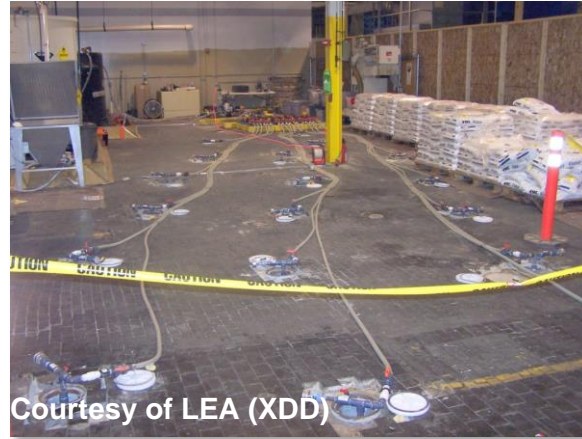
Injection/Recirculation via fixed wells
