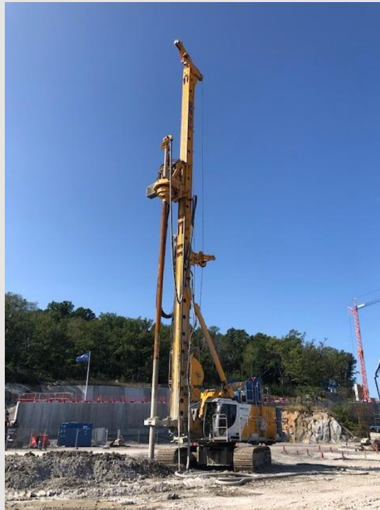
Klozur® SP, cement and water applied using large diameter auger
