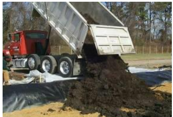
Figure 1: Placement of soil into treatment cell
