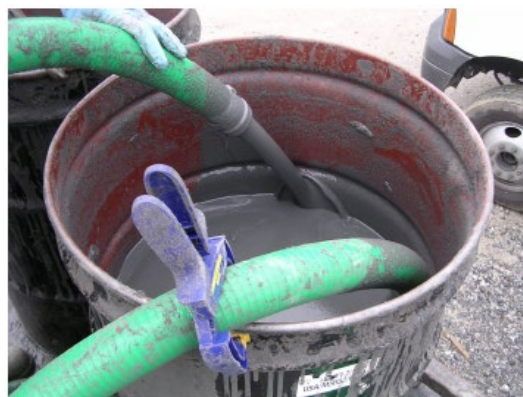
Figure 8. Mixing of EHC slurry using recirculation
