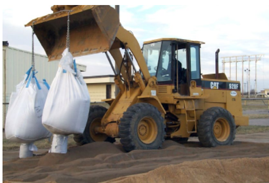
Figure 3. Dry mixing of EHC (provided in sacks) and sand
