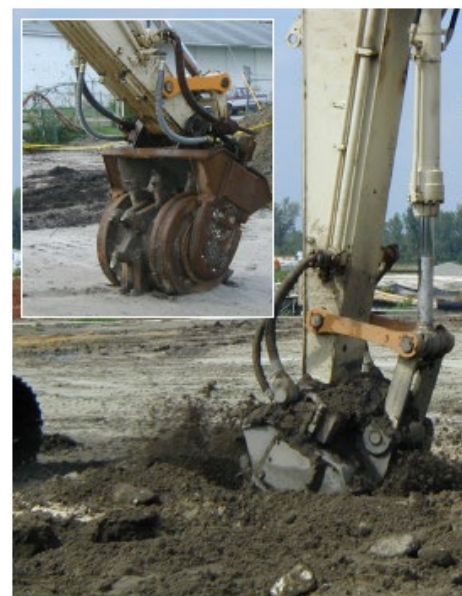
Figure 4. Deep soil mixing using a Lang Tool
