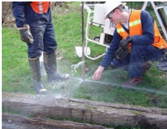
Figure 5. Injection tip with horizontal direction low pressure demonstration with water
